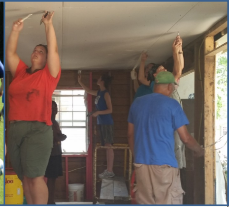
Lanesville Home Renovation Service Project
